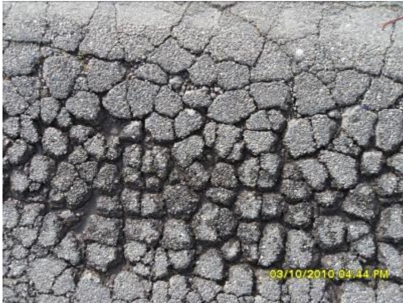
Reconstruction – The Street has a PCI of 17 (Close Up View)
